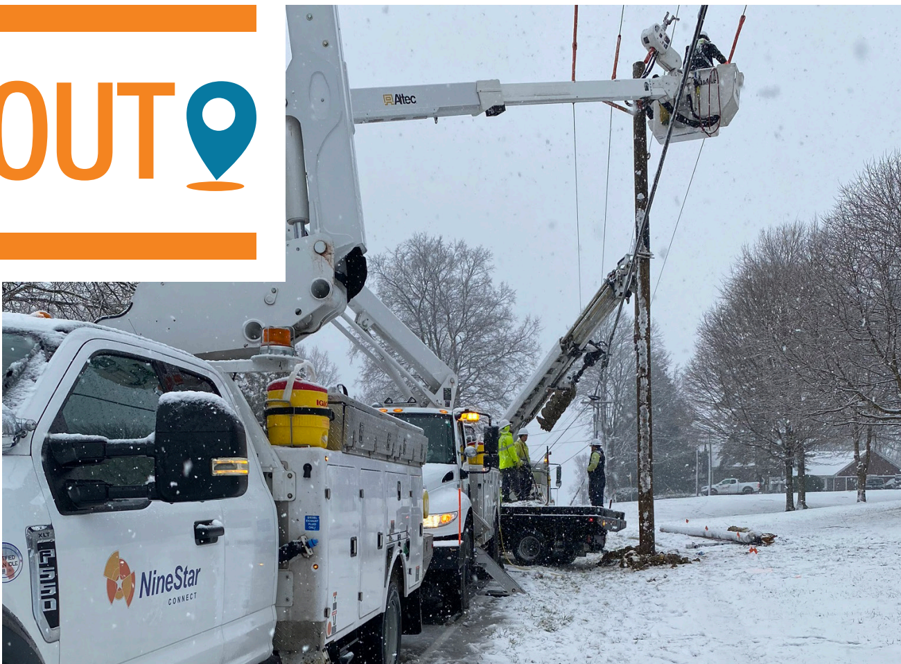
Line crews replacing a pole hit by a vehicle on 600 E.
